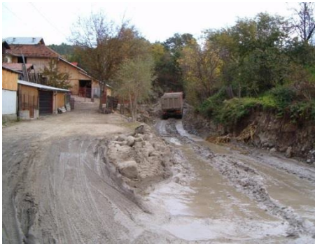
Figure 9 – in the village, the operations are started,
