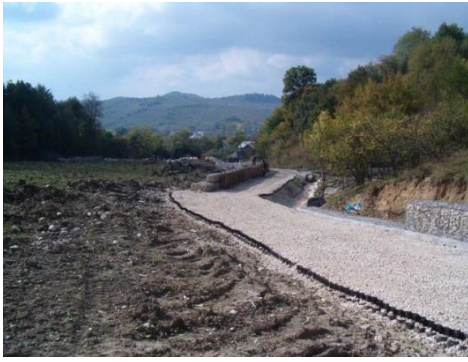
Figure 15 – the access way, built directly on slip,
