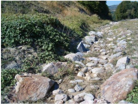
Figure 17 – surface water drainage channel built with natural materials,
