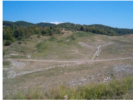
Figure 18 – "Y" shaped drains in the quarry,
