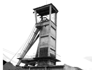
Fig.3. Hoist tower „ Auxiliary shaft “
