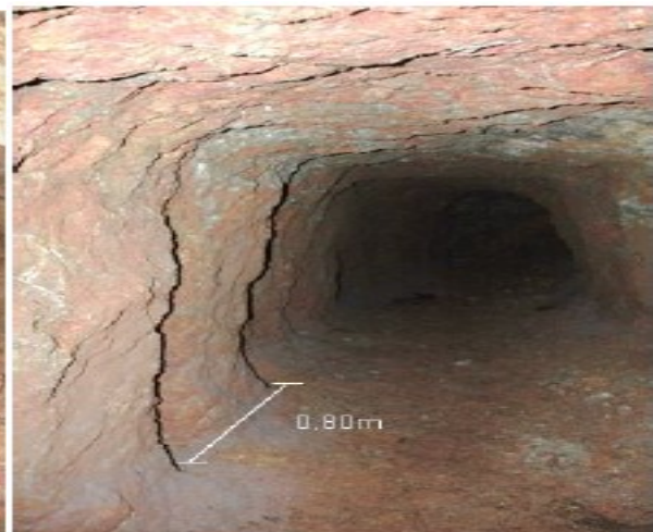
Figure 2.1.3-1: Crosscut A03, without Wall Collapsing
