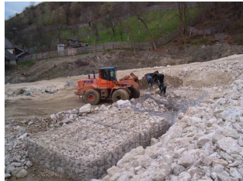
Figure 14 – gabions, in the downstream of the drainage wedge prism,
