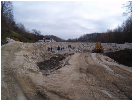
Figure 11 – in the downstream of the wedge prism, during construction,
