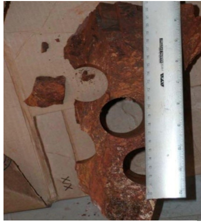
Fig. 2.3-2: Disintegrated Block after Drilling of the Test Samples
