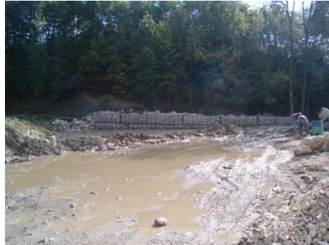
Figure 12 – the squeezing process, at the contact between the drainage wedge prism and slipping material,
