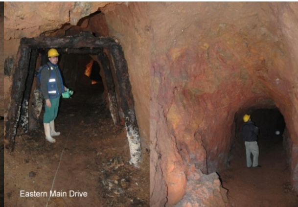
Figure 2.1.2-1: Eastern Main Drive with Roof Collapsing Features
